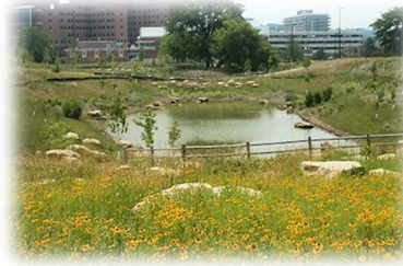
The constructed wetland basin included as part of the Art & Architecture storm water management system.
