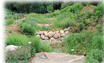
Vegetated swale with built in check-dam structures located at the University of Michigan Arboretum.
